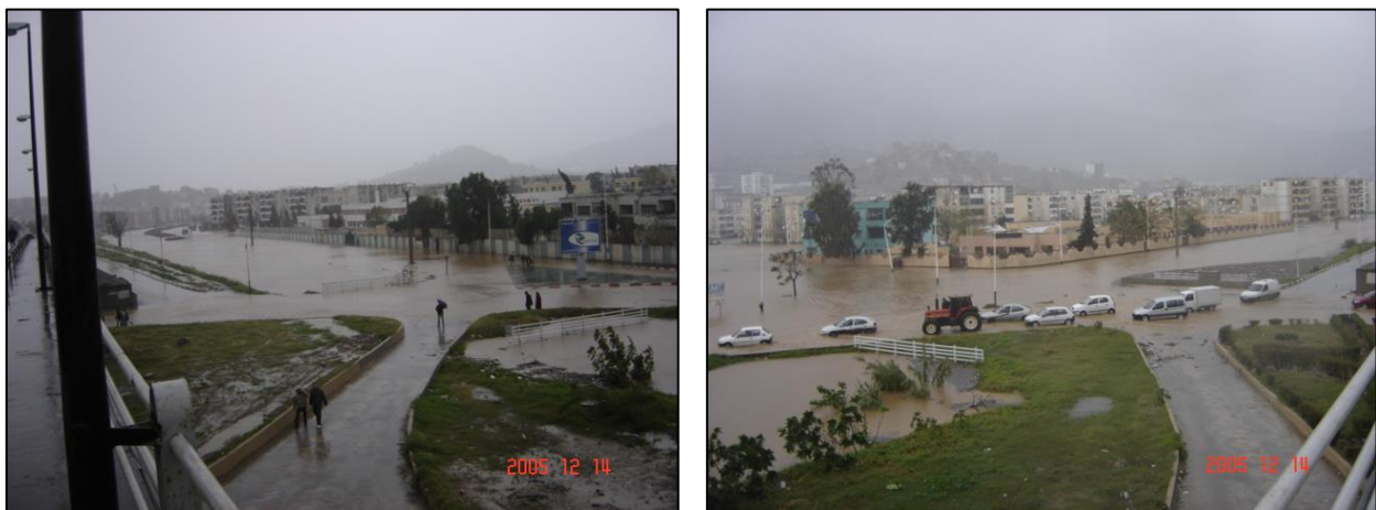
Figure 20: Overflowing of the belt canal (Bouhdid valley) event of 12, 2005.
