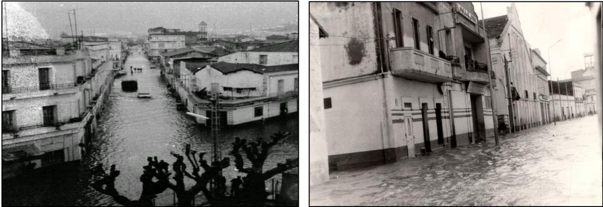
Figure 19: Floods of November 1982 in the city of Annaba.
