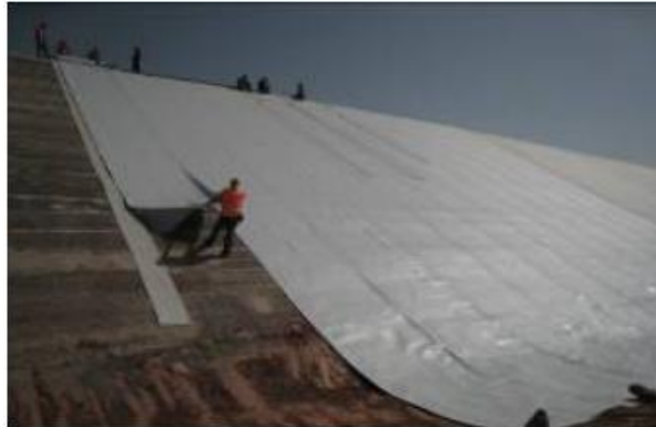
Figure 1.8: Pose de géomembrane (Barrage de Sar Cheshmeh, Iran)
