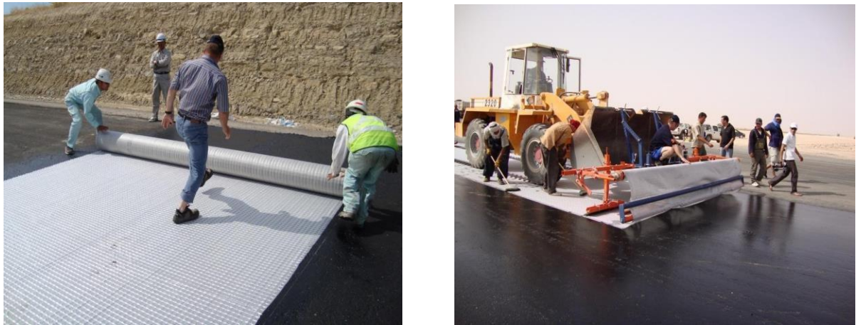
Figure II. 12 Renforcement des talus
