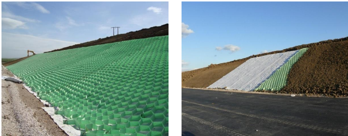
Figure II. 9 Protection Anti-érosion (Autoroute Est/Ouest)
