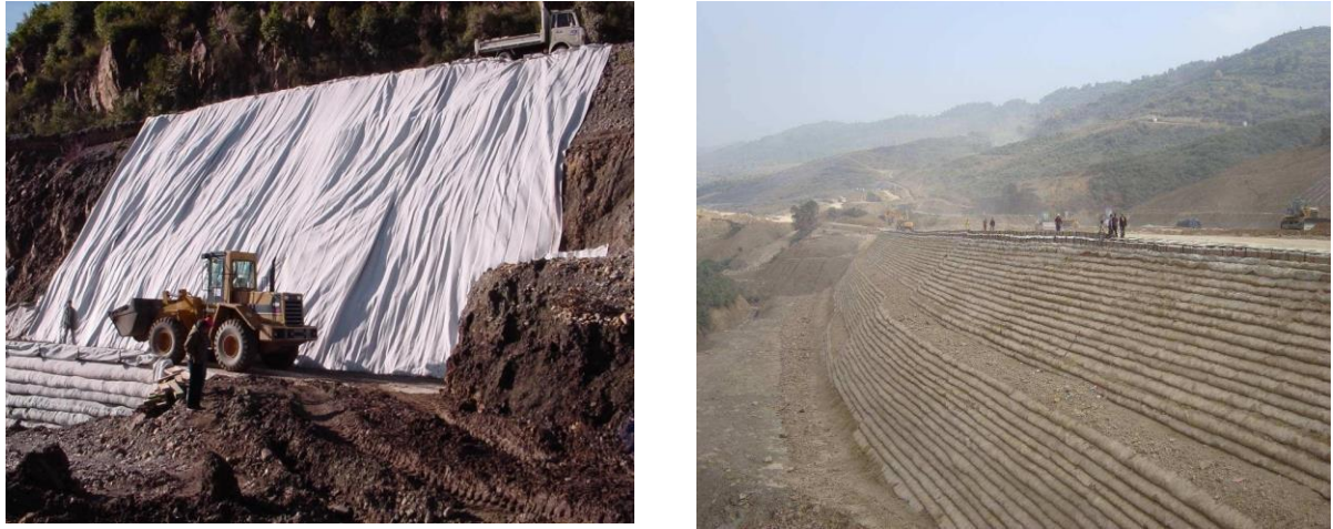
Figure II. 10 Renforcement des talus
